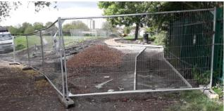
Unfortunately delays to tarmac supply meant that the surfacing of the path could not be done as planned to allow it to open. Rather than the delay the works to the track it was decided (given the dry conditions) to provide a temporary access across the grass and part of the turning circle while the works progressed.
