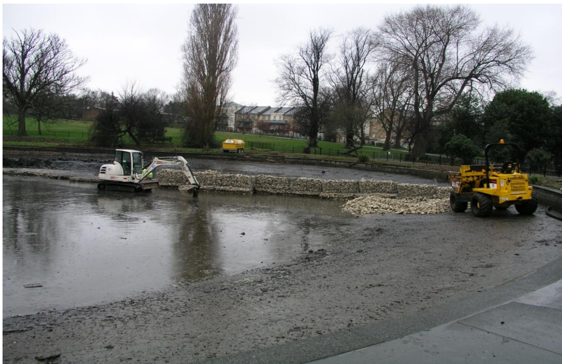
Photograph 8 – Gabion cages to create shallow areas for planting
